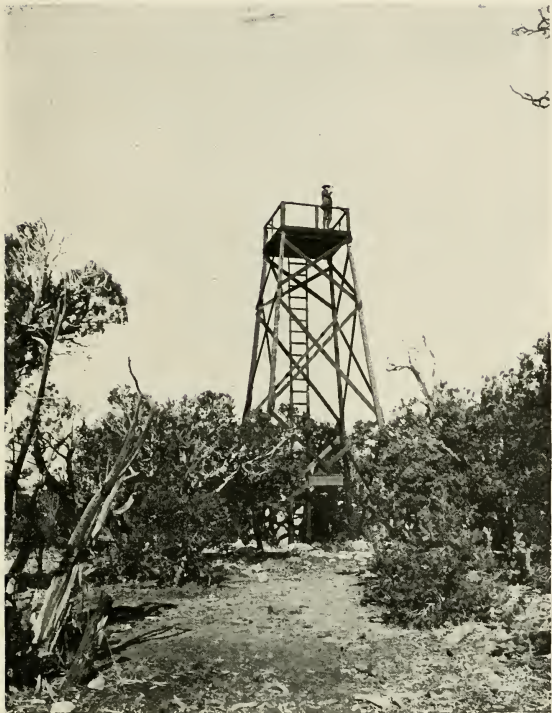
FIG. 62.—A Watch Tower in the Tusayan National Forest, Arizona.
